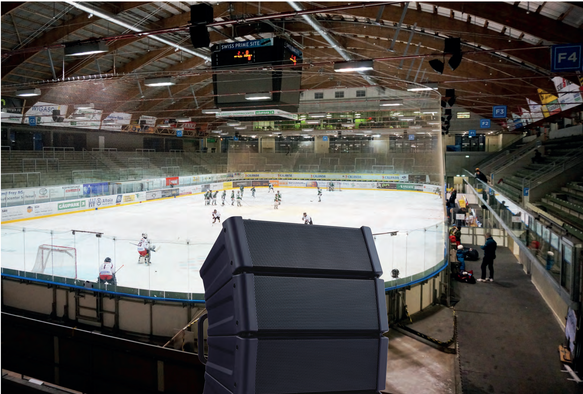
The professional PA in the renovated ice rink in Olten, Switzerland, is realized with Variable Compact Array Speakers HX-5. Low frequencies are supported by FB-120 subwoofers.
